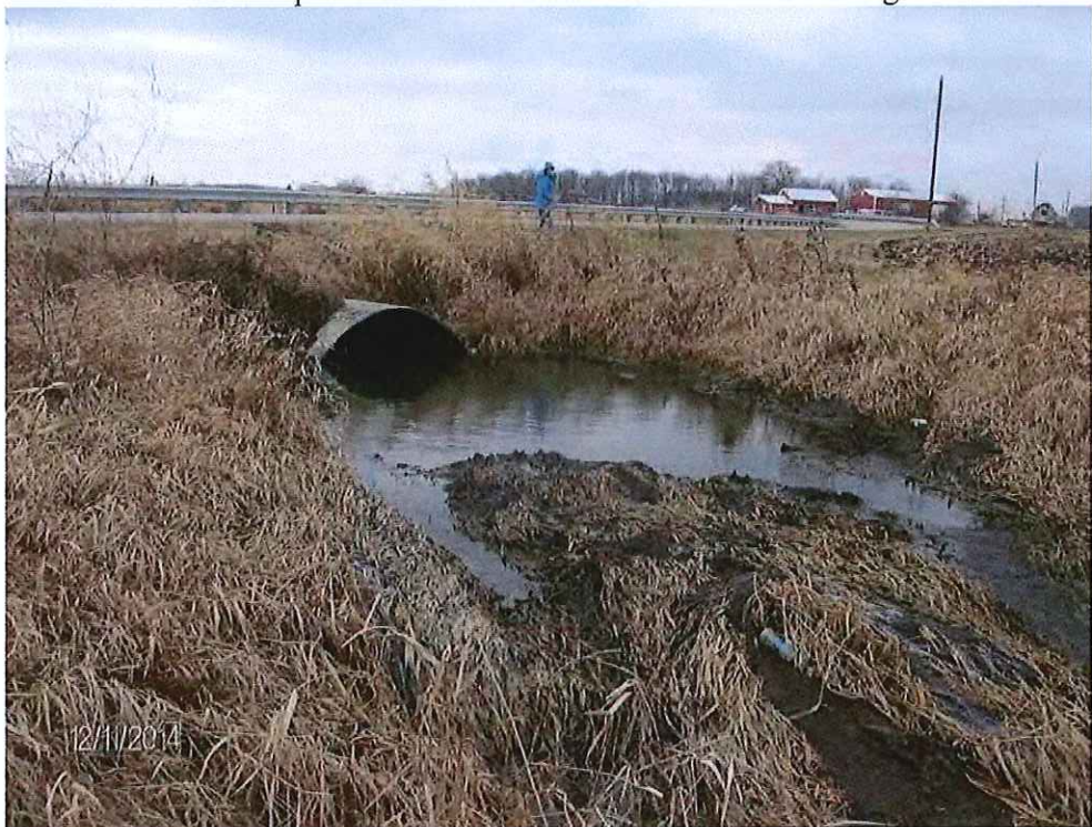
P28: Downstream Face of Upper 266 th Street Crossing
