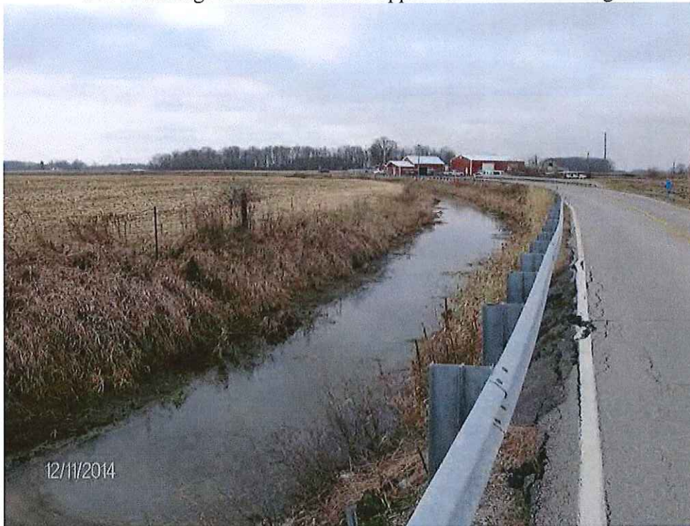
P30: Looking Upstream from Upper 266 th Street Crossing
