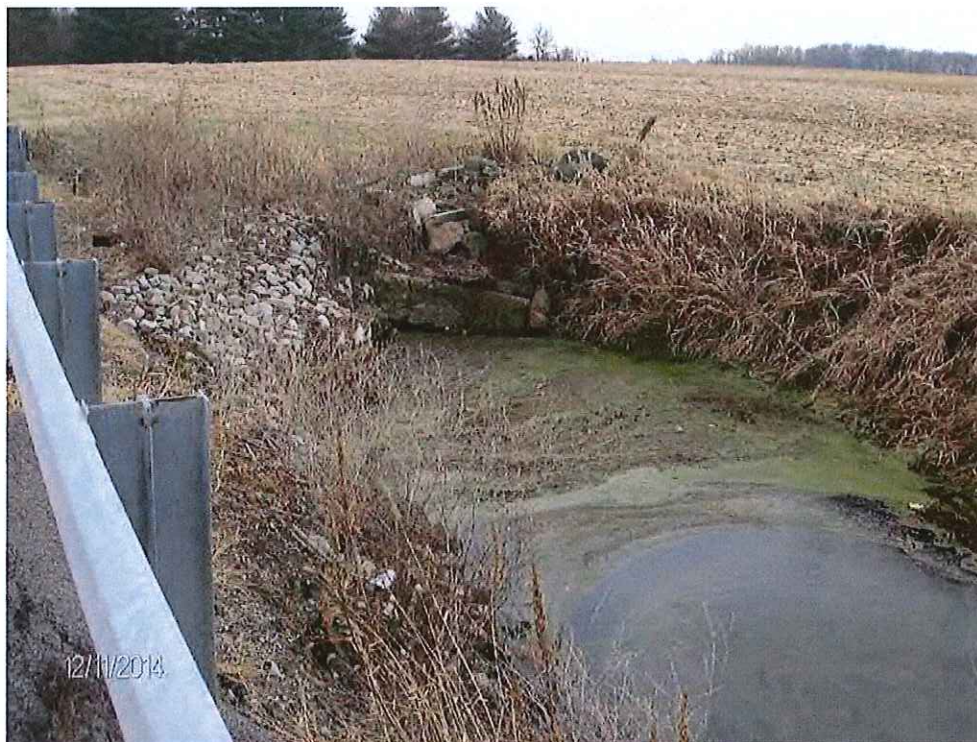
P31: Upstream Face of 266 th Street Upper Crossing
