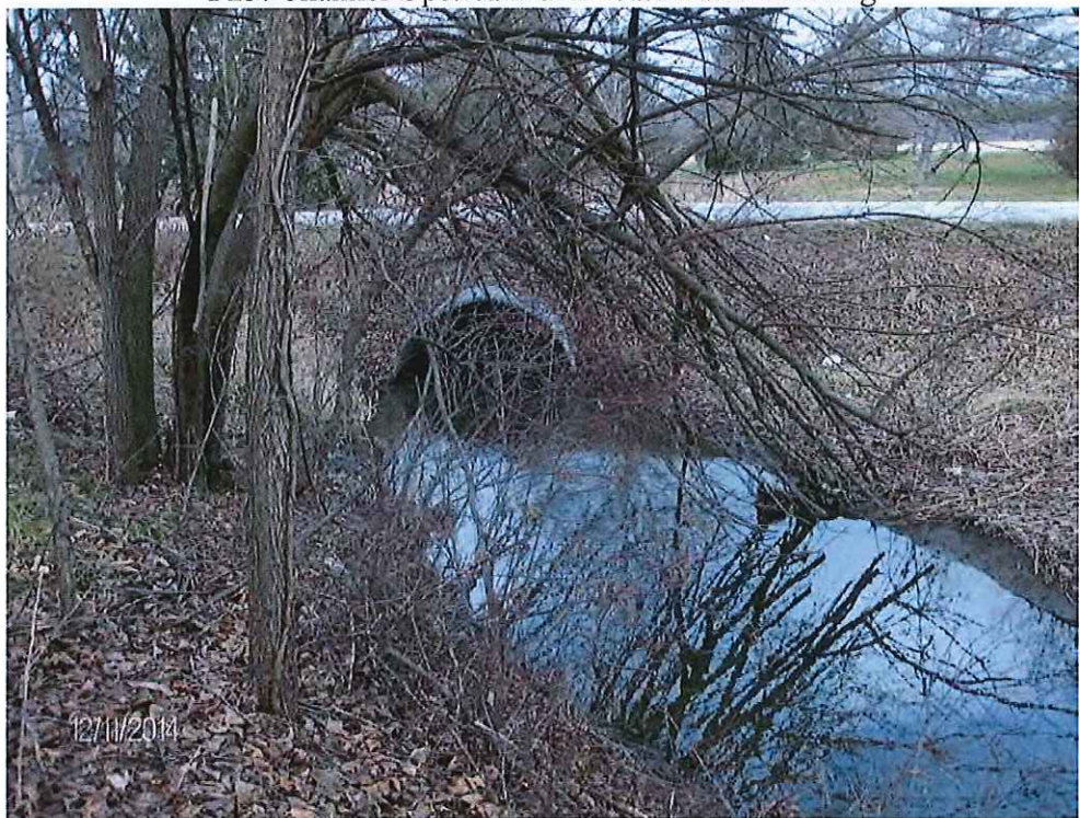
P24: Downstream Face of Middle 266 th Street Crossing
