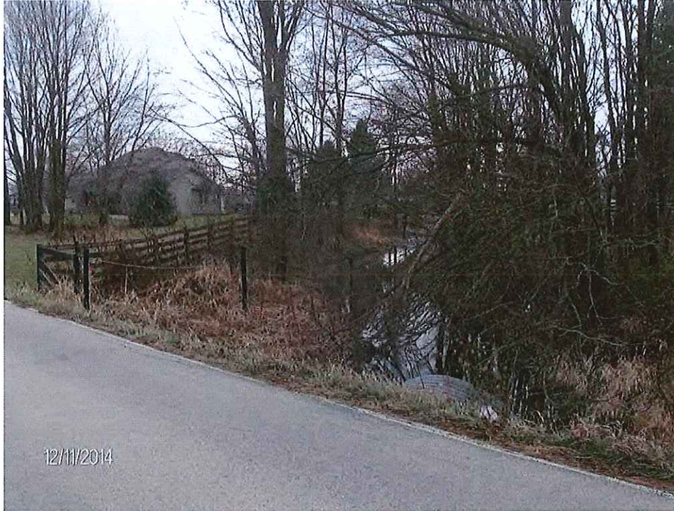
P25: Looking Downstream from 266 th Street Middle Crossing
