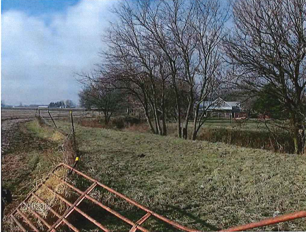
P21: Channel on Stepp Property (Station 100+00)
