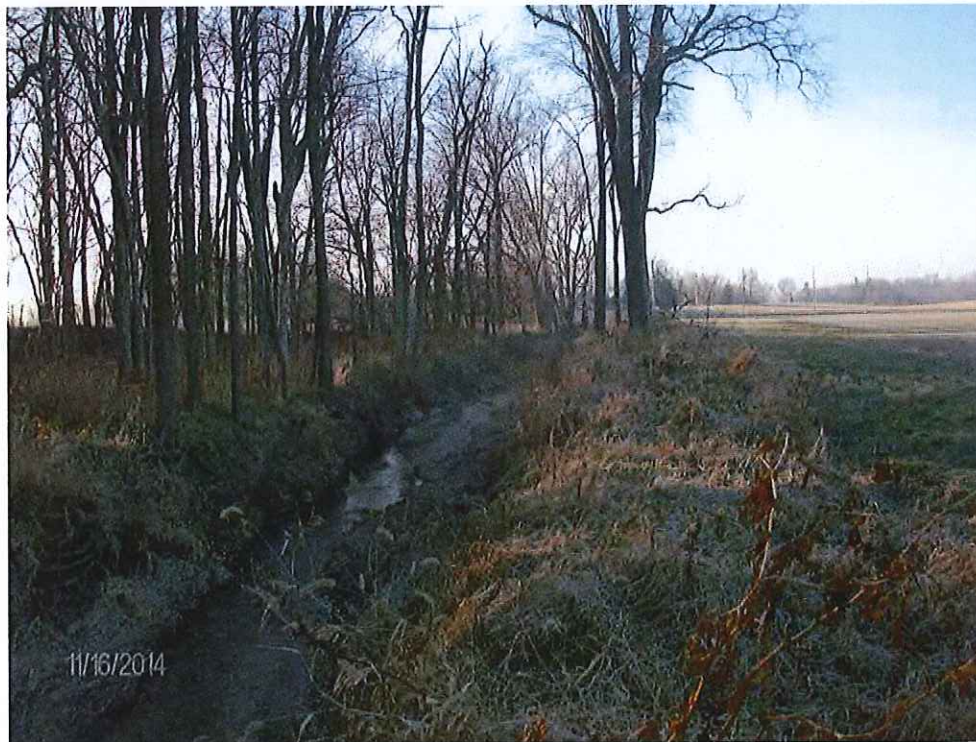
P2: Channel Downstream of 276 th Street (Looking upstream)
