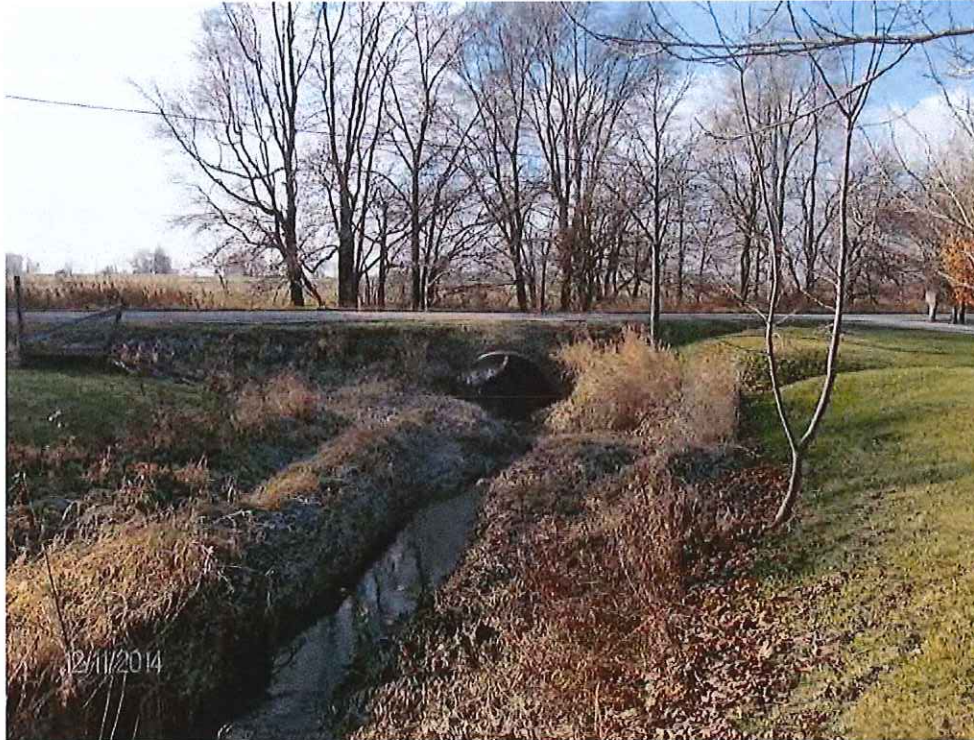
P17: Downstream Face of Downstream 266 th Street Crossing
