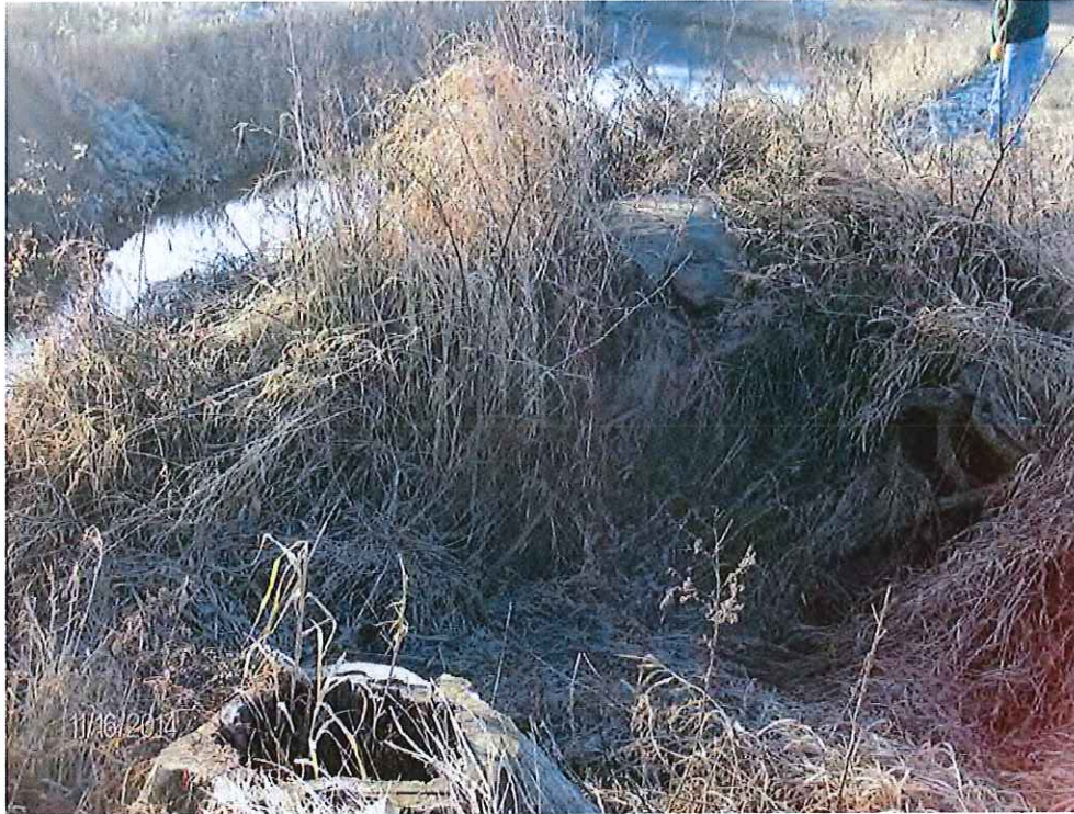
P3: Overbank Erosion at Station 6+00 (Left Side)
