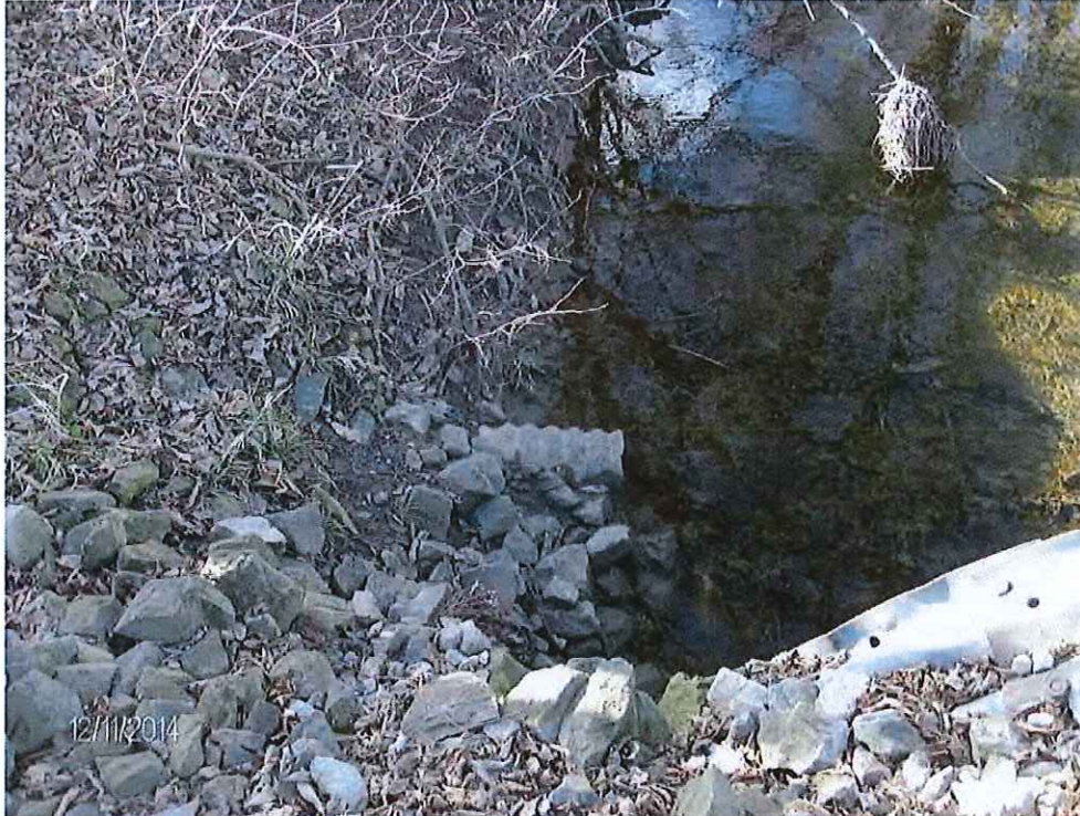
P19: Submerged Outlet just Upstream of 266 th Street (Station 93+31)
