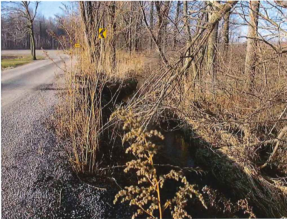
P8: Ditch Adjacent to Salem Road
