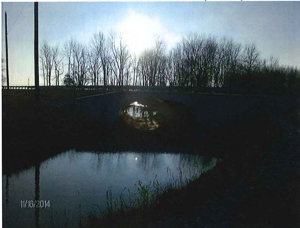
P4: Bridge Under 276 th Street
