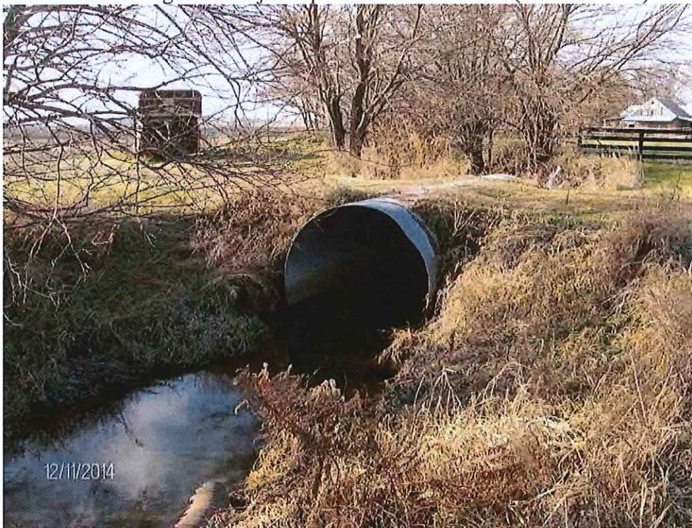
P20: Private Crossing on Clark Property (Station 98+00)
