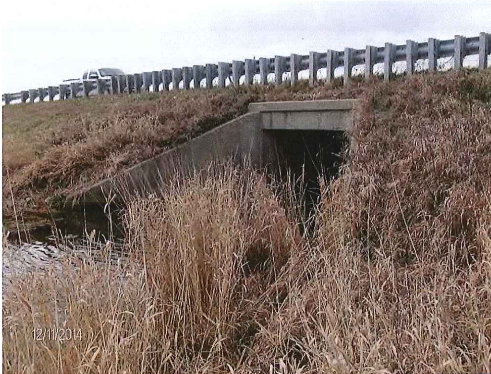
P33: Downstream Face of U.S. 31 Crossing
