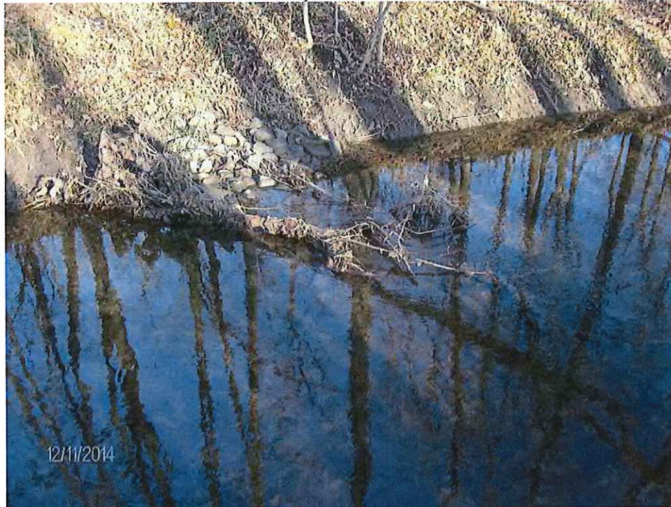
P10: Existing Ford Crossing on Duvall Bond & Harris LLC Property
