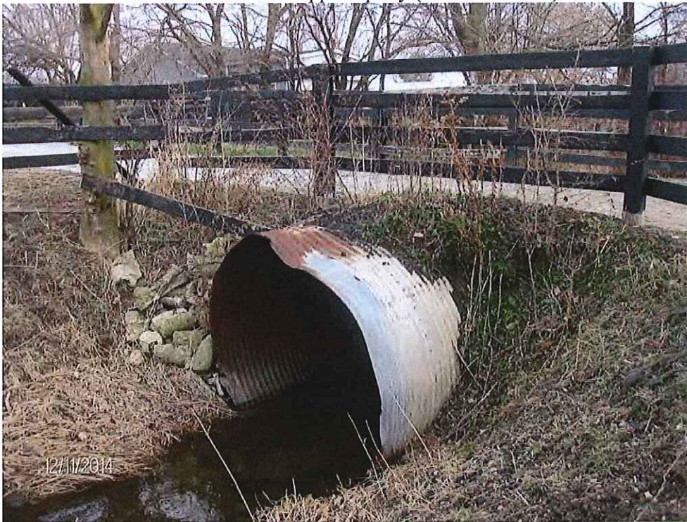
P22: Private Crossing on Bales Property (Station 104+50)
