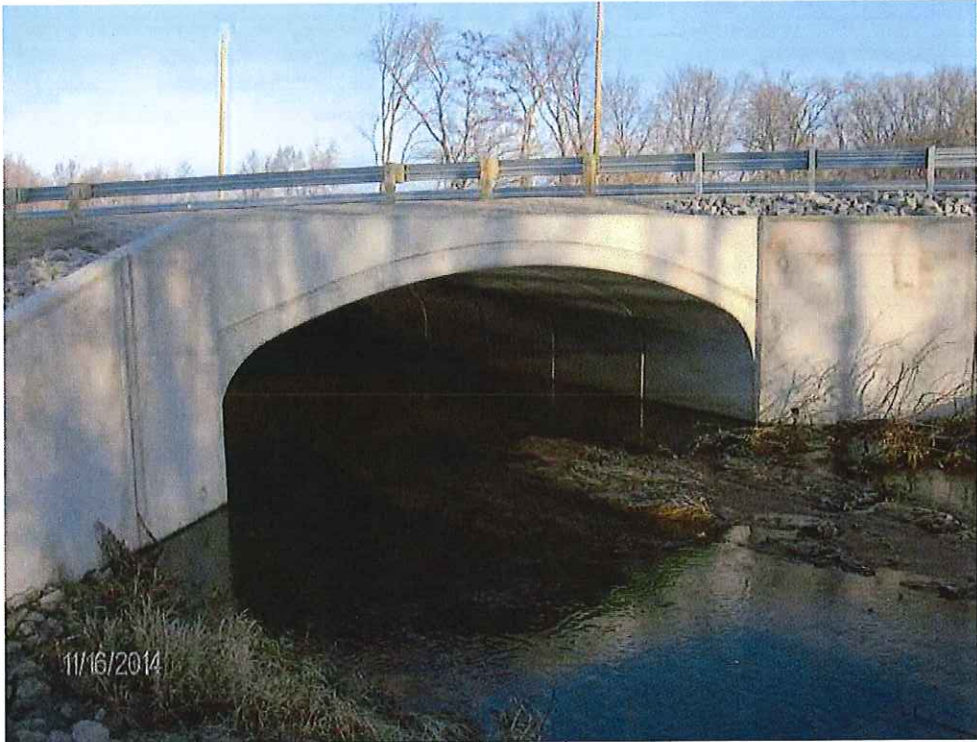
P5: Upstream Face of 276 th Street Bridge
