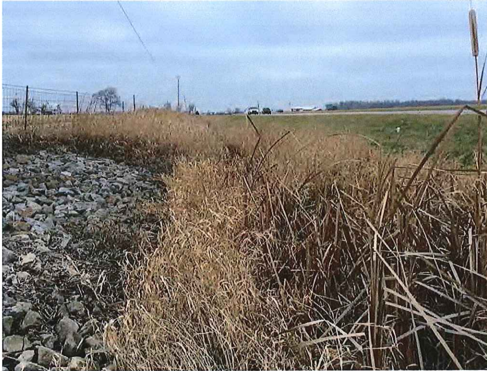
P37: Looking Downstream from Tile Outlet (Beginning of Open Drain)
