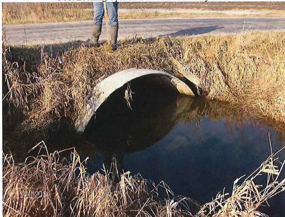
P12: Downstream Face of Anthony Road Culvert
