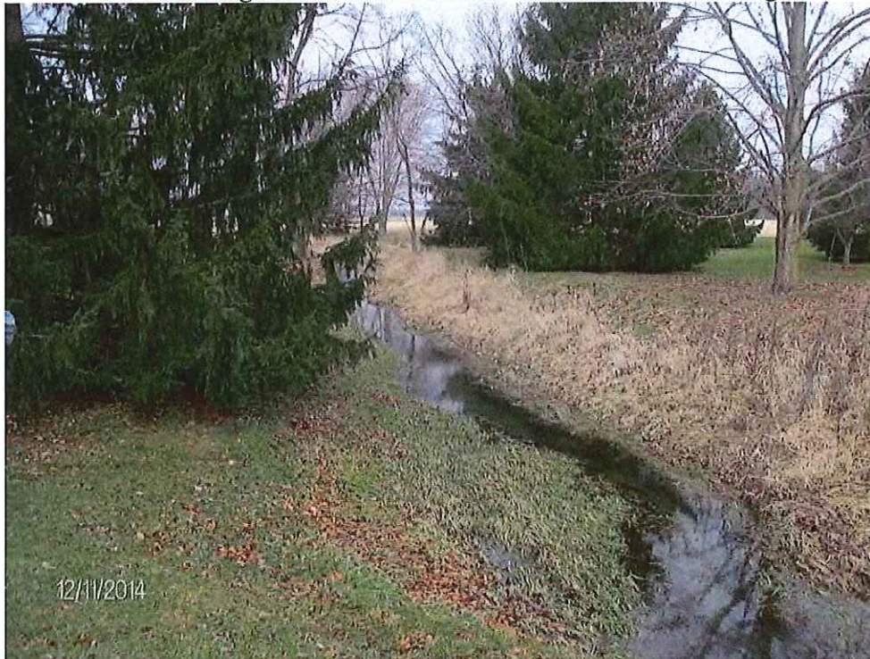
P26: Looking Upstream from Middle 266 th Street Crossing
