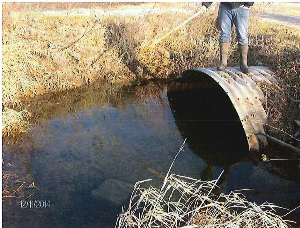
P13: Upstream Face of Anthony Road Culvert
